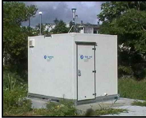
STATION URBAINE LAMENTIN
