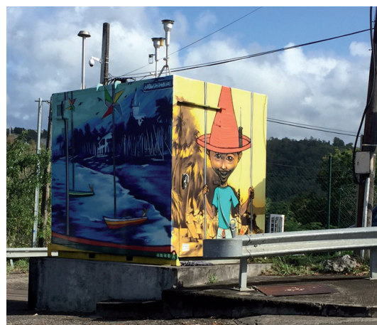
Figure 14. Station urbaine de Schoelcher
