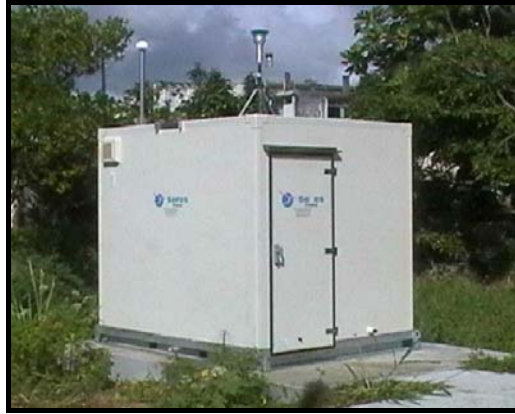
STATION URBAINE LAMENTIN
